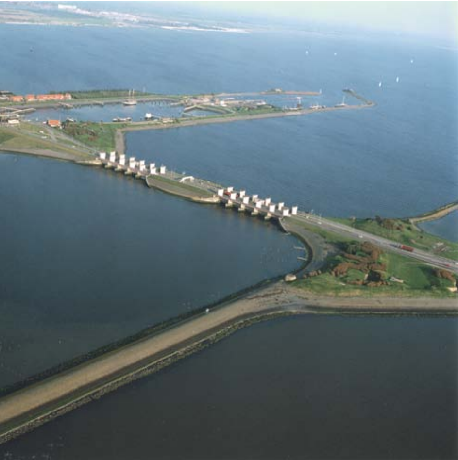
Lorentzsluizen, a complex of locks near Kornwerderzand, Friesland, in the Netherlands. The locks are part of the Afsluitdijk, a dike that dammed the Zuiderzee in 1932 to create both arable land and IJsselmeer, a freshwater lake.
