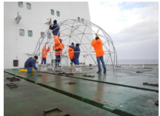
Fig. 2: Setup of the Domo-Tent-Structure (Photo Ulrich Freier, AWI).
