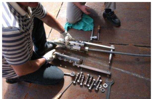
The disassembled cable termination. (photo: Saad El Naggari)
