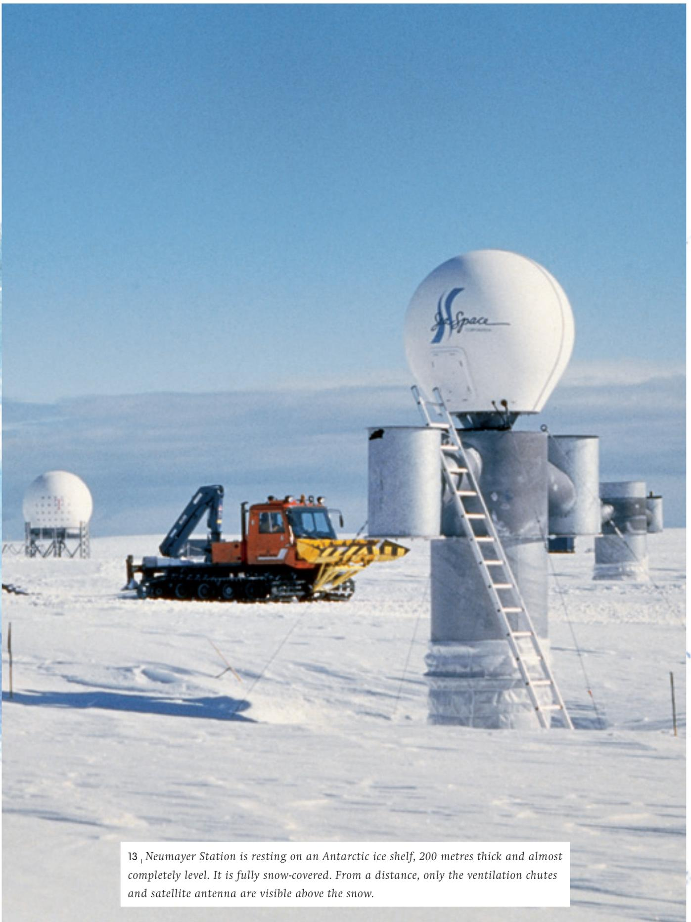
13 , Neumayer Station is resting on an Antarctic ice shelf, 200 metres thick and almost completely level. It is fully snow-covered. From a distance, only the ventilation chutes and satellite antenna are visible above the snow.
