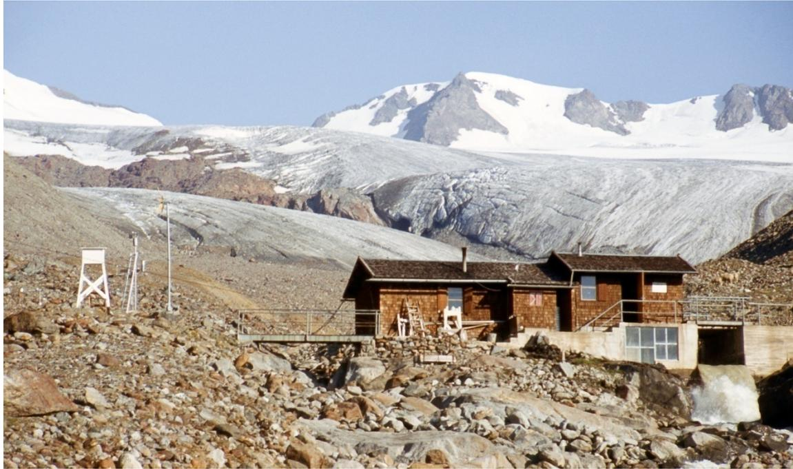
Fig.2: Hydrological part of the Vernagtbach station; from left to right: Stevenson screen and Wölfler anemometer (the same as in Fig.1), wind generator for power supply, gauging station Vernagtbach. The photograph was taken by Hans Oerter in September 1979.
