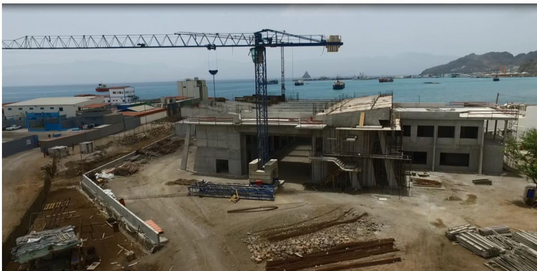
Fig. 1: Construction site of the Ocean Science Centre Mindelo (Photo: Björn Fiedler)
