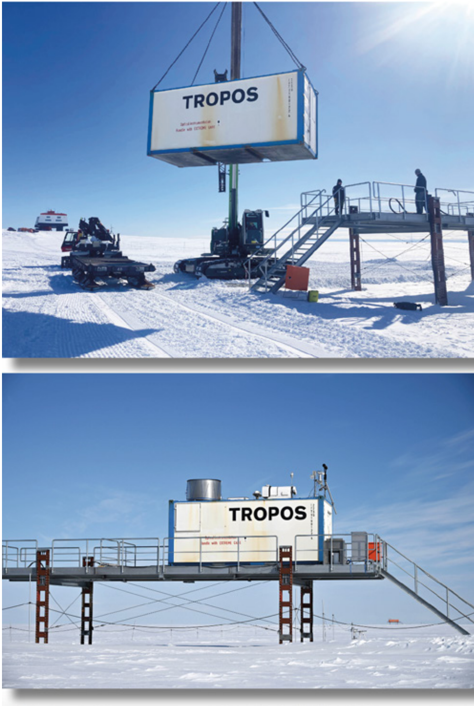
Fig. 4.20.1: Top (a): The TROPOS OCEANET-Atmosphere container is placed onto the platform 400 m south of the station. Bottom (b): The final setup where all instruments are installed on top of and next to the container
