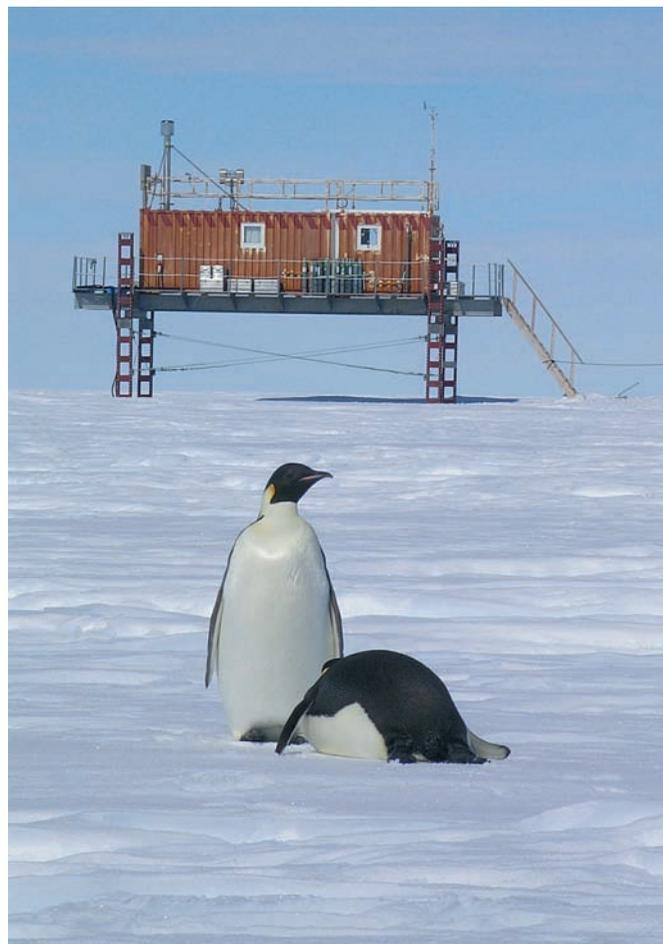
**Fig. 10:** The Neumayer air chemistry observatory after ten years of continuous operation in January 2005. Note the seriously rusted container casing.
