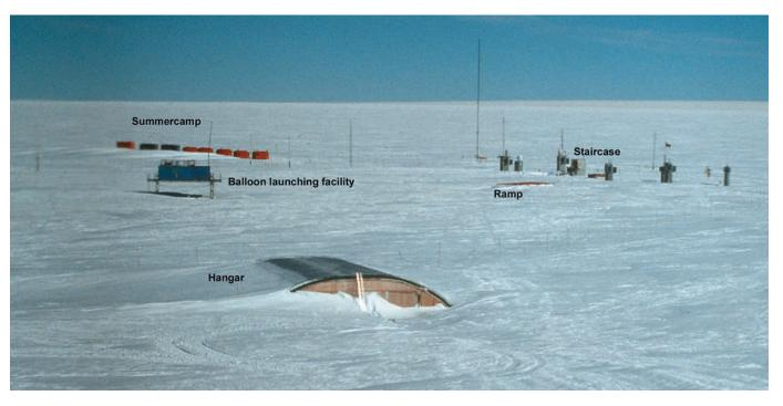
Fig. 6: Area view of Georg von Neumayer Station (GvN) in 1989. In front the aircraft hangar almost completely covered by snow. Entrance towers, exhaust pipes and antenna domes in the right centre mark the position of the GvN structure beneath the snow. Behind the balloon-launching container (centre left) of the meteorological observatory the red emergency huts are visible in the background (AWI).
