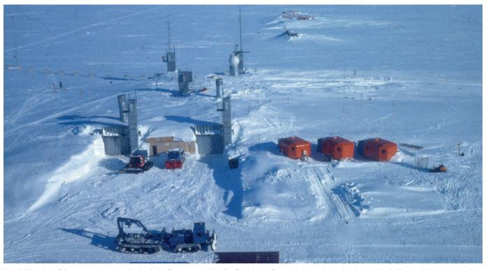
Fig. 2: Situation of Georg von Neumayer Station in its first season 1981. The first phase of construction at the station is completed. The steel tubes are completely covered by snow. During the second construction phase during austral summer 1981/1982 the cross tube serving as a vehicle garage will be annexed (D. Enss / Polarmar).
