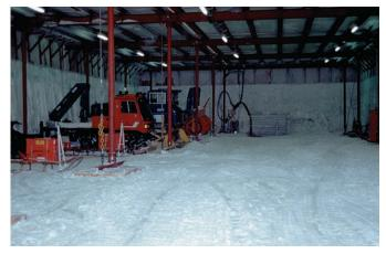
**Fig. 15:** View into the vehicle garage of Neumayer Station II (NM-II) in 1999. The garage is built into the firm with a new type of roof construction, which is regularly corrected according to the snow accumulation and surface.
