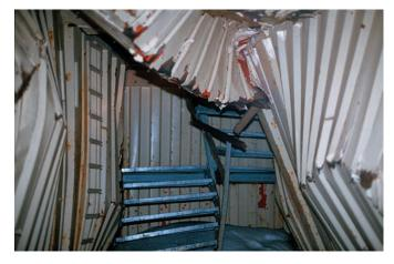
Fig. 9: Georg von Neumayer Station (GvN) in 2000. Eight years after abandonment of the station the staticase shows strong demolition by ice pressure.
