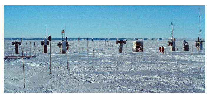
Fig. 7: Georg von Neumayer Station (GVN) in 1989. Staircases, ventilation shafts and antennas roughly mark the position of the station beneath the snow surface. The four emergency exit towers indicate the ends of the tubes.
