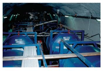
Fig. 13: View into the fuel storage of Neumayer Station II (NM-II) in 1999 showing six inter-connected diesel tanks with a total capacity of 130,000 l.
