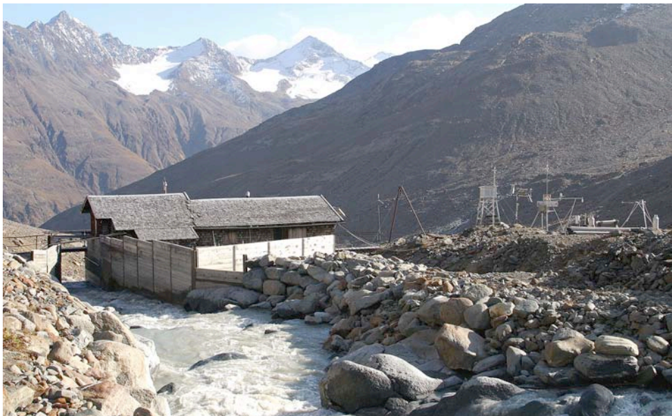
Figure 1: Gauging station “Vernagtach” at 2640 m a.s.l. with the wooden walls to protect the station from high flows, with the climate station on the right. (Photo taken 30 September 2003 by L. Braun).
