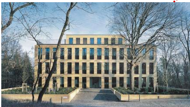
A45: AWI building
