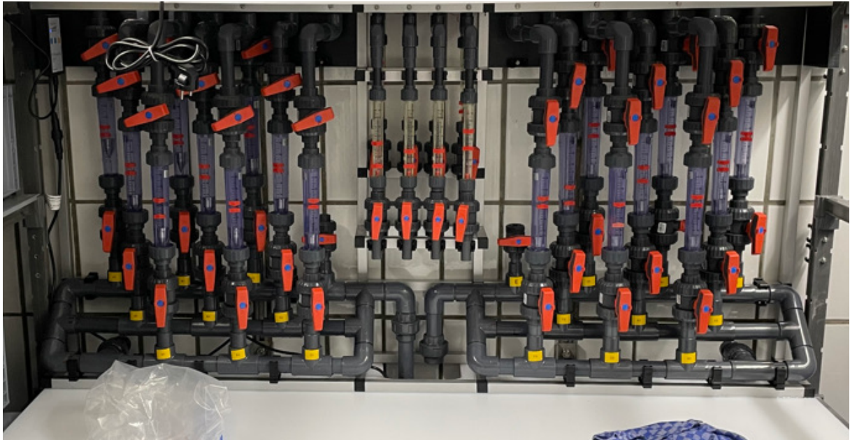
Figure 11: Central control panel (“The Organ”), to control the flow-through of each broodstock tank individually. © Jan Lammers
