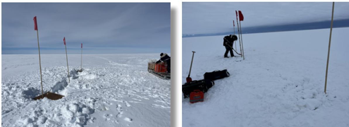
*Fig. 4.12.1: Maintenance and new deployment of the ApRES system controller (center pit) and two frame antennas (front and back pits) of the site after completion of the new deployment on 2 January 2023, with the system buried at about 20 cm depth below the current surface (left picture) and system controller (two flags in center) and each frame antenna (left and right flag) covered with wooden boards. The Iridium antenna is mounted on the bamboo pole with black tape (right picture).*
