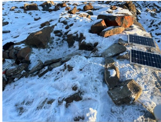
Fig. 5.2.1: PEAR station. Zarges box on the left, two solar panels and GNSS antenna on the right
